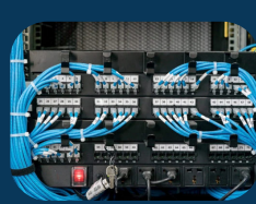
CABLING , DRESSING & LABELING
